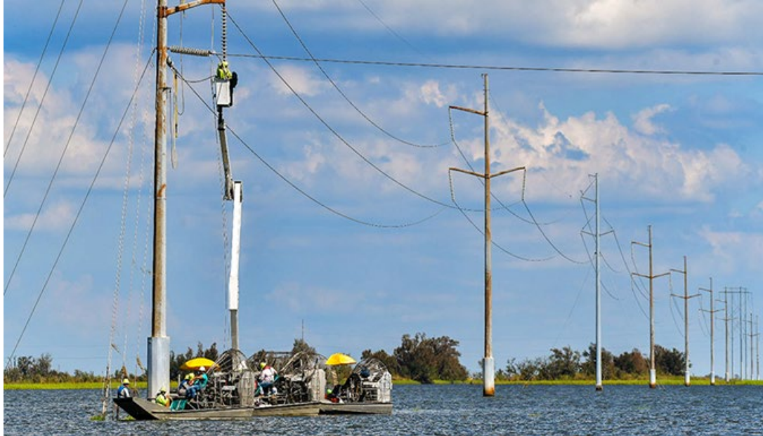
Lineman working to restore power after Hurricane Francine; Source: Entergy
