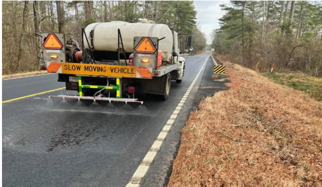
Pretreat of roads across Louisiana has begun ahead of winter weather Photo credit: Louisiana DOTD on Facebook
